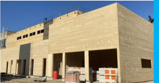
New Thermal Treatment project in Amiens
